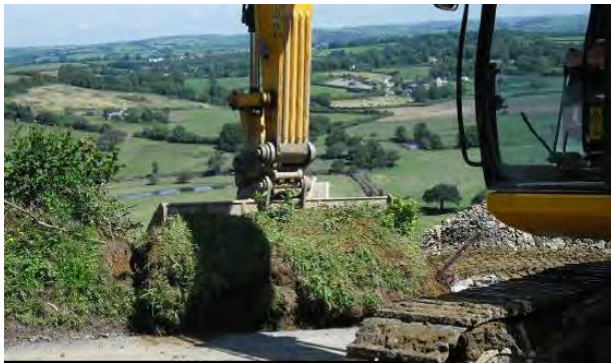
Removing slab of hedgerow ground flora
